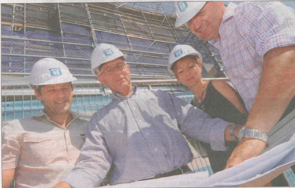
CHECK IT OUT: Quarterback Group project managers Peter Stemm (left) and Mark Roy (right) inspect the Aspex Gladstone plans with architect Walter Betten (centre left) and interior designer Amanda Taylor (centre right). Picture by CHRISSY HARRIS
