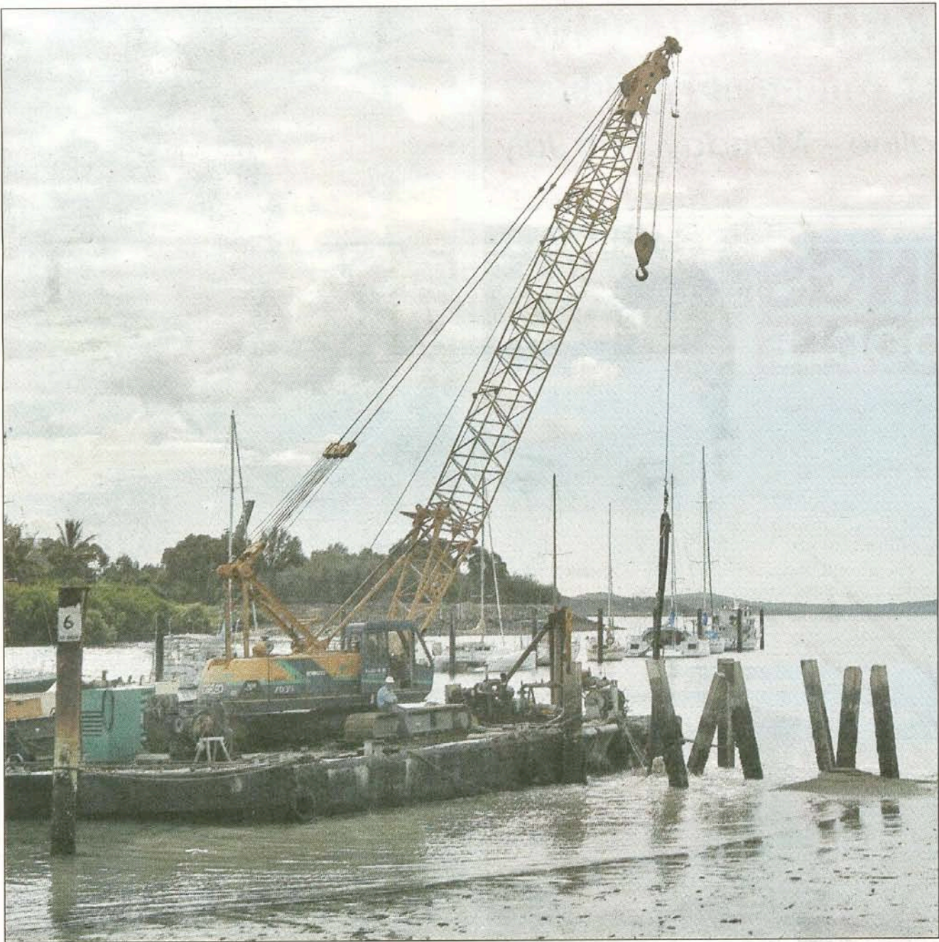
BIG JOB: Removal of the old pilings from O'Connell Wharf.
