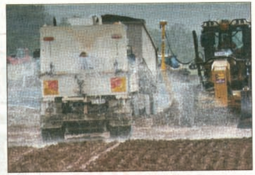
SOLID: Water trucks help prepare the foundations for the new runway.
