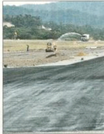
TARMAC LAID: Keeping the dust down. Picture: CHRISSY HARRIS GLA_airp250510-9
