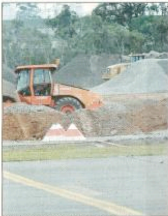
STONE'S THROW: Work progresses. Picture: ALEX NEWTON GLA_airp250510-22
